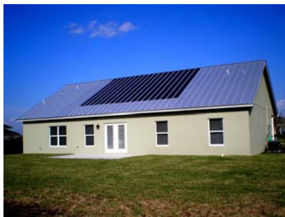
2.5 Kw Residential Uni-Solar system
